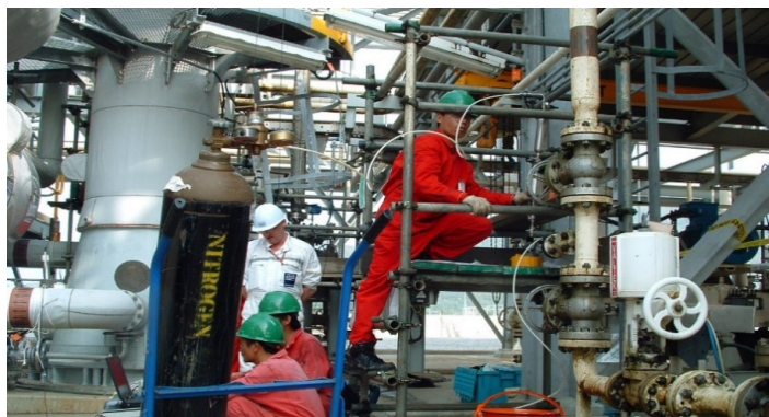
Radiotracer for Leak detection in gas treatment plant
